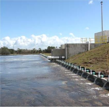
*ATS™ surger and distribution systems provides flow at linear hydraulic loading rates of 10 to 20 gal lf<sup>-1</sup> min<sup>-1</sup>*
