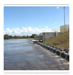
ATS<sup>TM</sup> surger and distribution systems provides flow at linear hydraulic loading rates of 10 to20 gal  $lf^{-1}$  min<sup>-1</sup>
